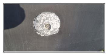
and to various overboard discharges by a clearly marked multi stranded earth wire of about 4mm square. The copper strip / bonding was examined as far as practicable limitations of access allowed and was found generally in a fair condition.
